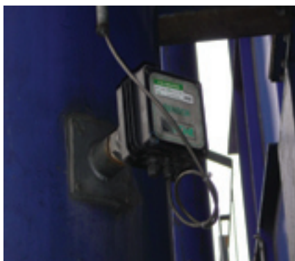
The interspace between Primary and Secondary HEPPA Filters monitored by an approved (MCERTS, TUV) Electrodynamic Sensor
