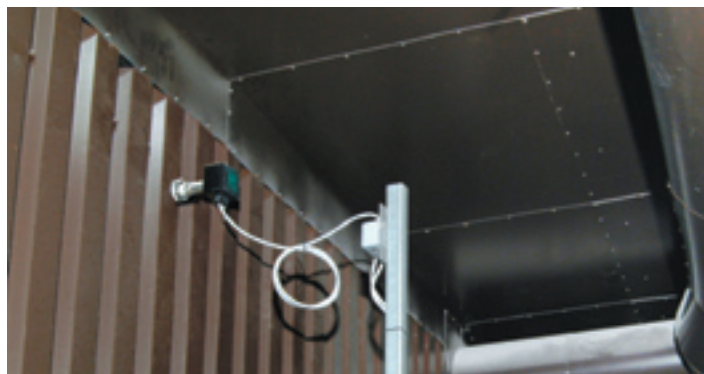
Electrodynamic sensor mounted in chamber wall
