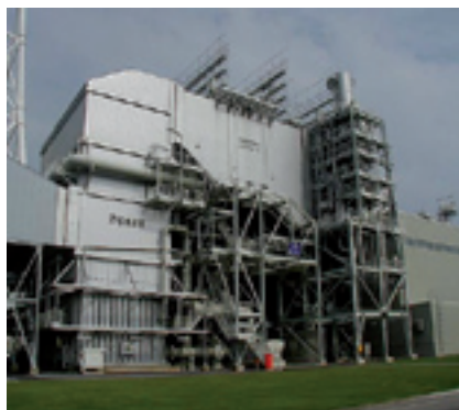
Flue Gas Desulphurisation Plant
