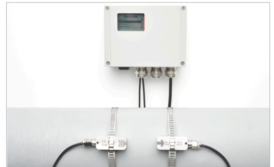
Two KATflow 100 flowmeters were then installed as part of a permanent metering and monitoring package
