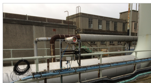
The installed KATflow 170 with stainless steel enclosure at ESSAR Oil
