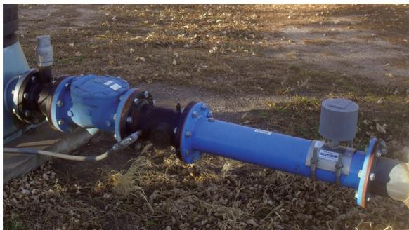
Figure 4: Mc Propeller Flow Meter With Integral Flow Straightener Installed At A Pump Station
