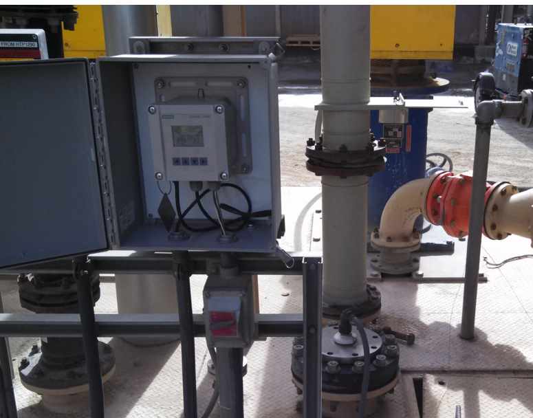
Commissioning the SITRANS LUT400 was very easy – with the controller's Quick Start Wizard, the new level measurement system was up and running in record time.
